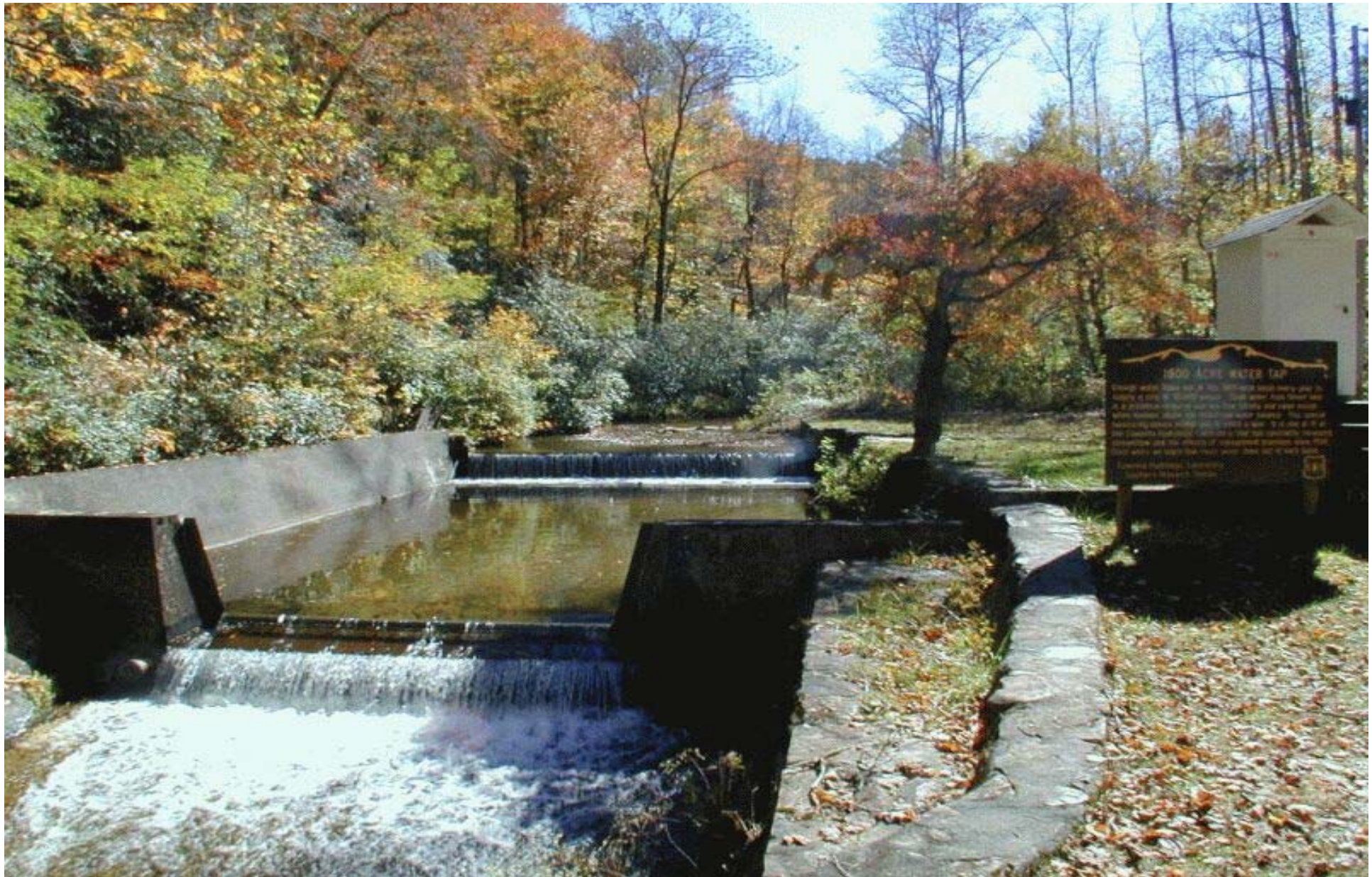
Ball Creek Weir - 2004
